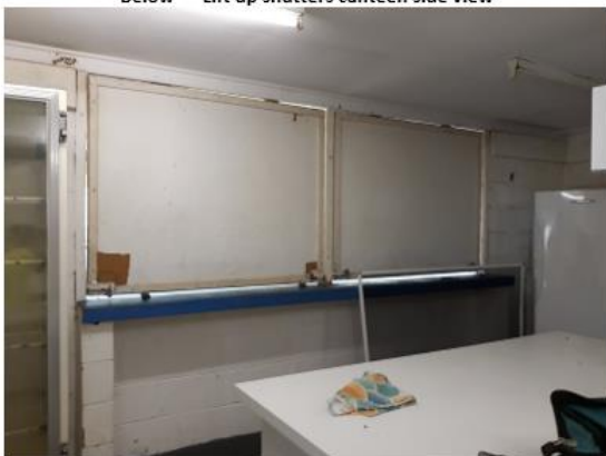
Below Lift up shutters canteen side view
